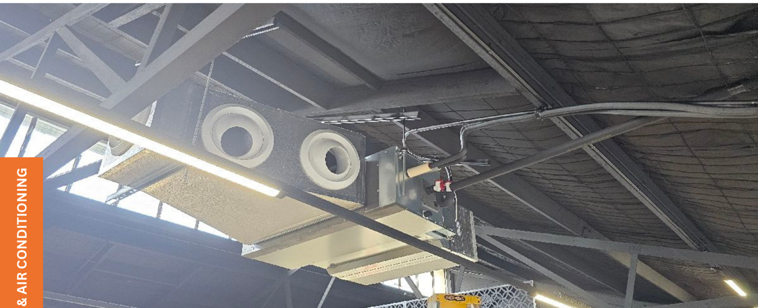
Image: 20kW Ducted Install - Fortitude Valley
